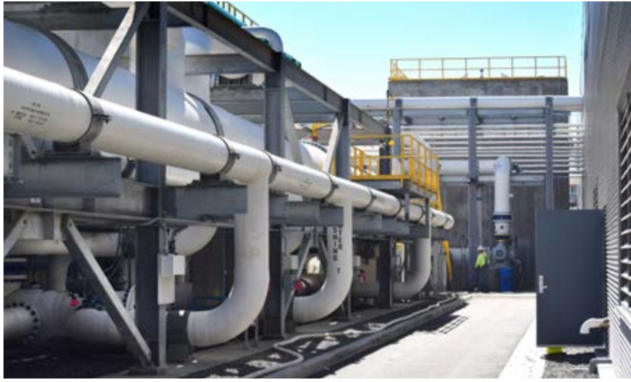
The Claude "Bud" Lewis Carlsbad Desalination Plant turns sea water into 50 million gallons of drinking water each day.
