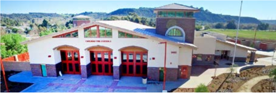
Fire Station 3 provides first responders with a modern building and expanded space to meet current and future public safety needs.
